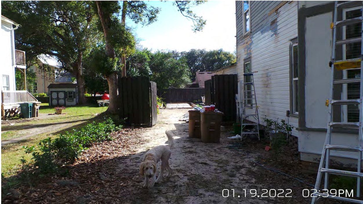
Photo 1: Photo of front of SE 726 SE 3 rd Street. Driveway will be install on left side of house.
